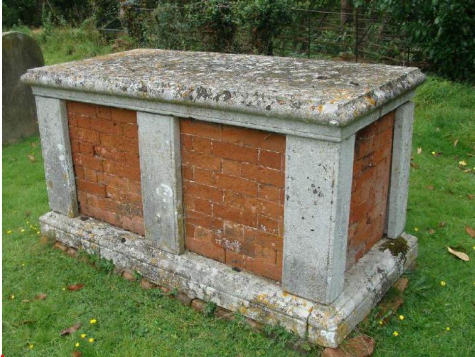
Picture 143 – One of many fine chest tombs in the churchyard, this one being of stone and rubbed brick.
