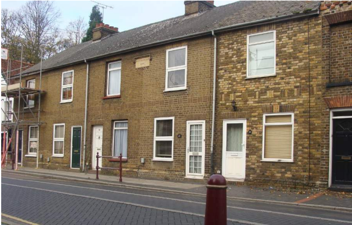
Picture 4. Various window and door types are uncoordinated on this terrace in the District.
