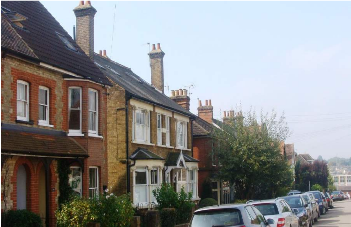
Picture 3. This photograph illustrates the various and generally unspoilt architectural detailing to the front elevations of dwelling houses within a street in the Bishop's Stortford Conservation Area.
