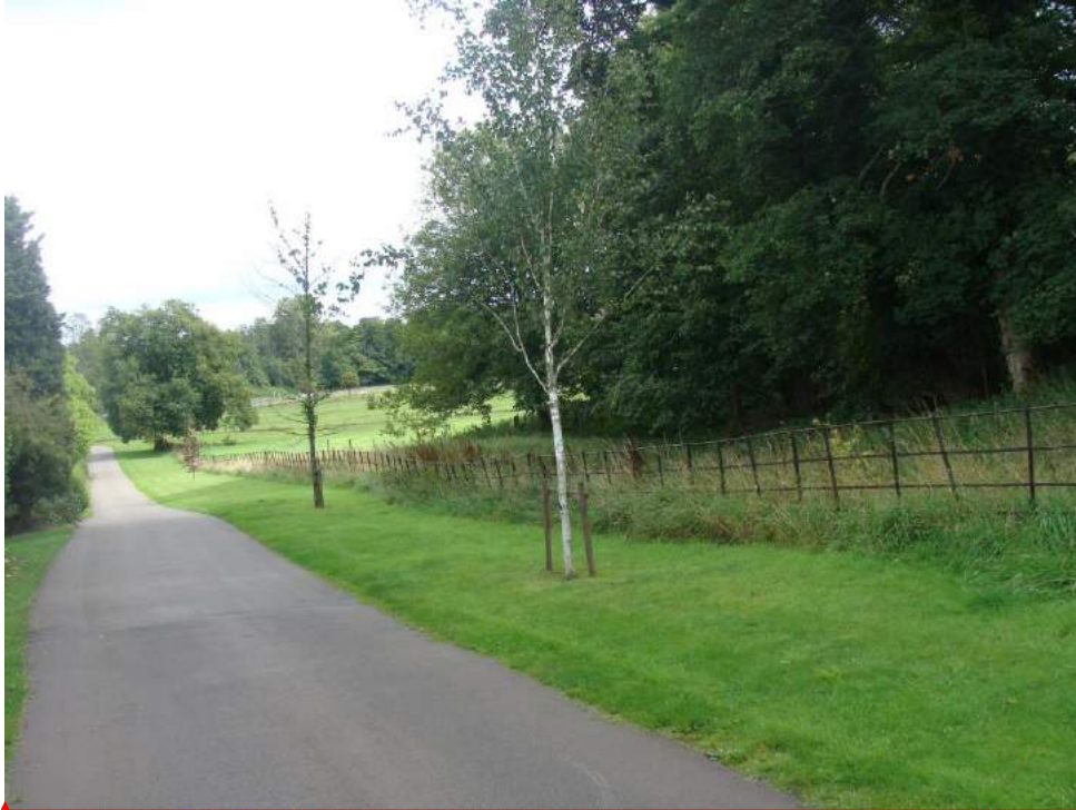
Picture 175 – 19 th /20 th century metal estate fencing of quality that adds to the rural qualities of the Conservation Area in this location and which should be retained.
